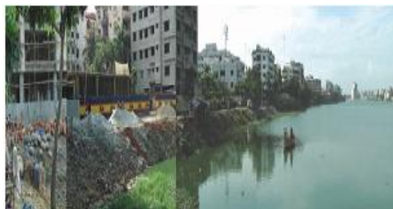
Damped Construction Materials
